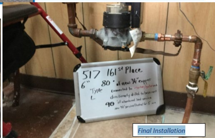
Drilling of Water Service
