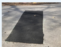
Permanent asphalt patching in the road.
